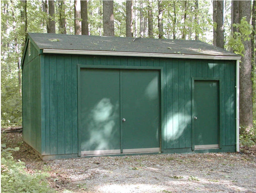
Figure 1. Building 112, the JHU/APL magnetism facility building.
