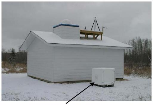
Observatory Equipment housed in Environmental Enclosure (the "hut")
